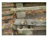
built have deteriorated. The area around the steps has been filled with years of soil driven by runoff. Foundations have shifted, and some of the steps are unstable. The concrete platform is showing its age and needs replacement as well.
