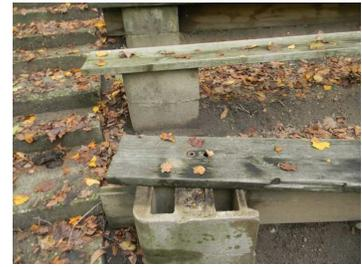
filled with years of soil driven by runoff. Foundations have shifted, and some of the steps are unstable. The concrete platform is showing its age and needs replacement as well.
